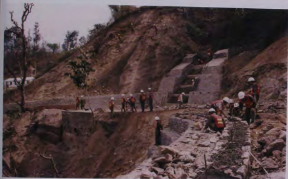
Exercise Holdfast , 1996, in East Nepal. 67 Gurkha Independent Field Squadron constructing a major culvert and a gabion retaining wall.
