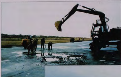
Crater repaired with AM2 by I Troop 59 Independent Commando Squadron.
