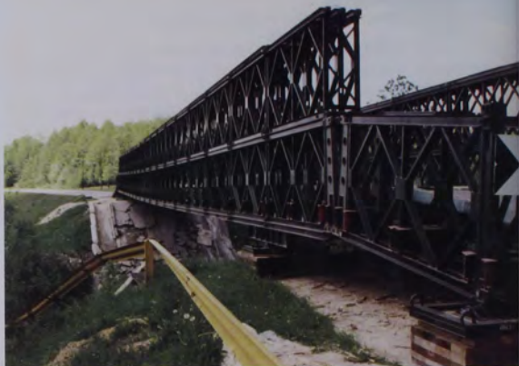
Above: Double Triple Bailey (Perie) Bridge near Sipovo.
