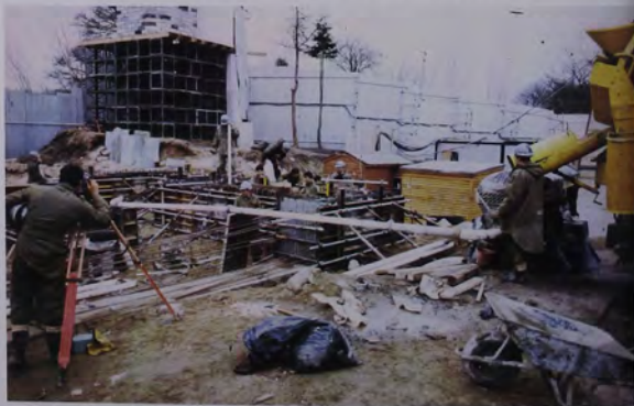
Above: Operation Amulet , 1987, Plumbridge, undertaken by 51 Field Squadron. The old RUC station before reconstruction. Below: Pumping concrete during construction.
