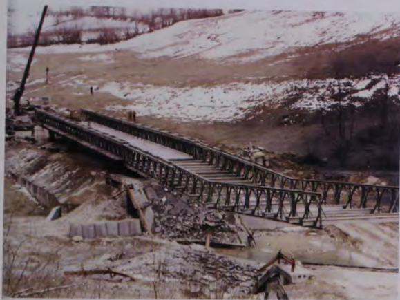
Above: The Class 70 Triple Single HGB built by 32 Armoured Engineer Regiment on Route Clog.
