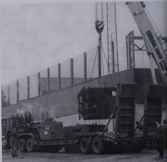
Above: Andersonstown RUC Station, Belfast. The super sangar/lowloader, linked to the rebuild after the 1983 VNIED. Opposite page: Design development after seventeen years.
