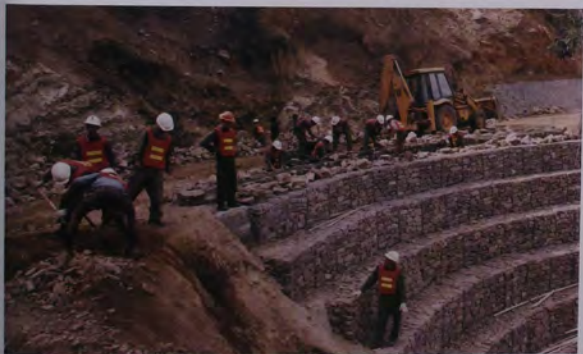
Exercise Holdfast , 1996, in East Nepal. 67 Gurkha Independent Field Squadron constructing a major culvert and a gabion retaining wall.
