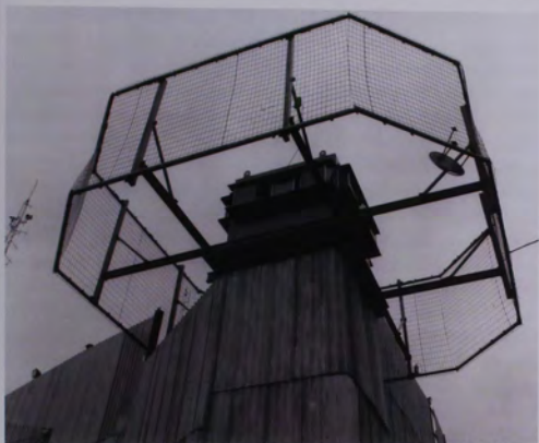
Above: Forkill sangar design. Below: Operations centre, showing sacrificial roof.
