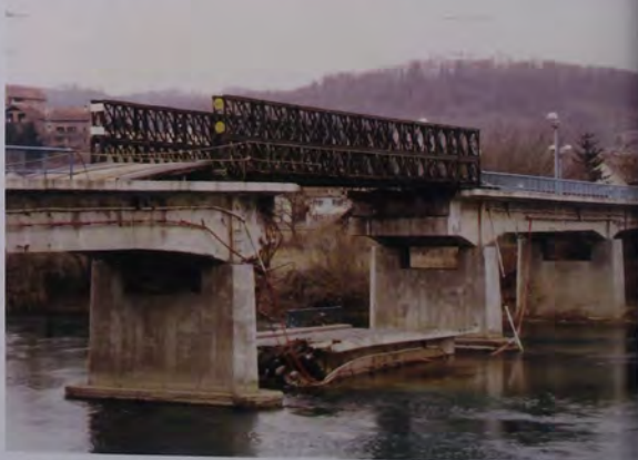
The Class 40 double-double Bailey built by 32 Armoured Engineer Regiment over the River Una for Czech deployment.
