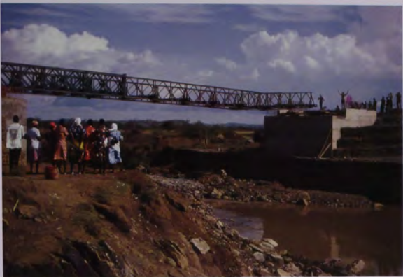
Above: The bridge being launched across the River Gucha.
