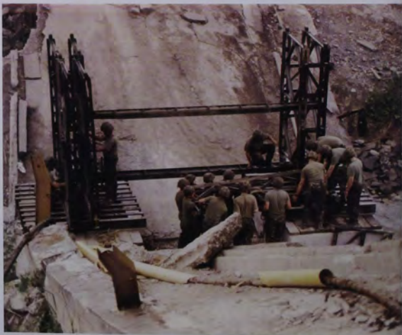
Below: Members of 32 Armoured Engineer Regiment building a pier under Perie Bridge.
