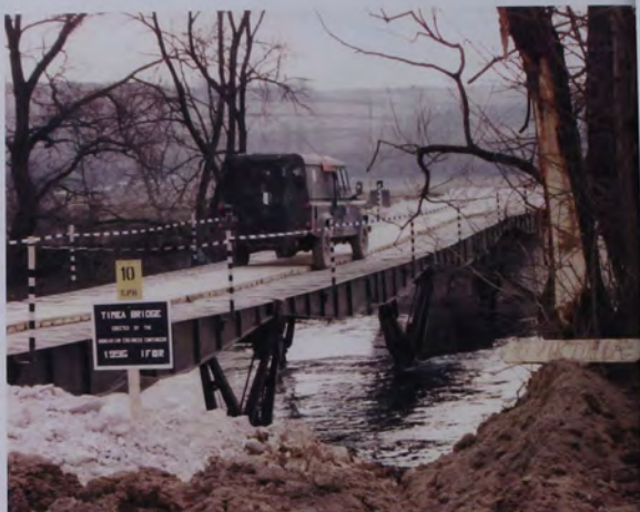
Above: 'Timea Bridge' – TMM erected by the Hungarian Engineers. Below: The Canadian Engineer's improvised bridge near Bihać.
