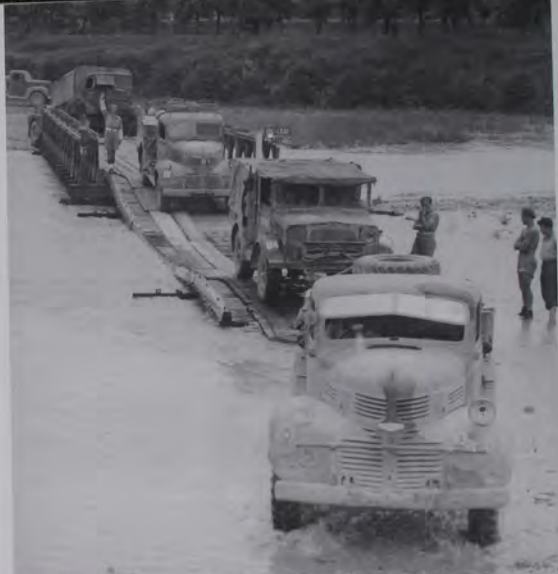
A column of trucks crossing a Bailey bridge over the Arno River, near Figline, 11 August 1944. Imperial War Museum, London
