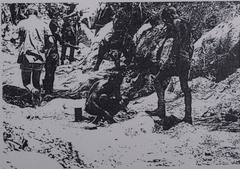
Below: Sappers prepare PE-4 charges for blasting to improve depth and gradient of channel to improve water flow.
