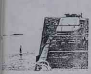
Portable compressor, an Ingersoll-Rand 600-cfm Gyro-Flo, supplied air for submerged rig. The top of the drill tower can be seen protruding from the water at the left.
