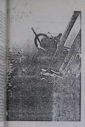
Diver on ocean floor (left and on cover) gets set to sink first of daily series of blastholes. Rubber hose to lead drift's compressed air exhaust bubbles out of diver's way was one modification required to adapt I-R drill rig for submarine work.
