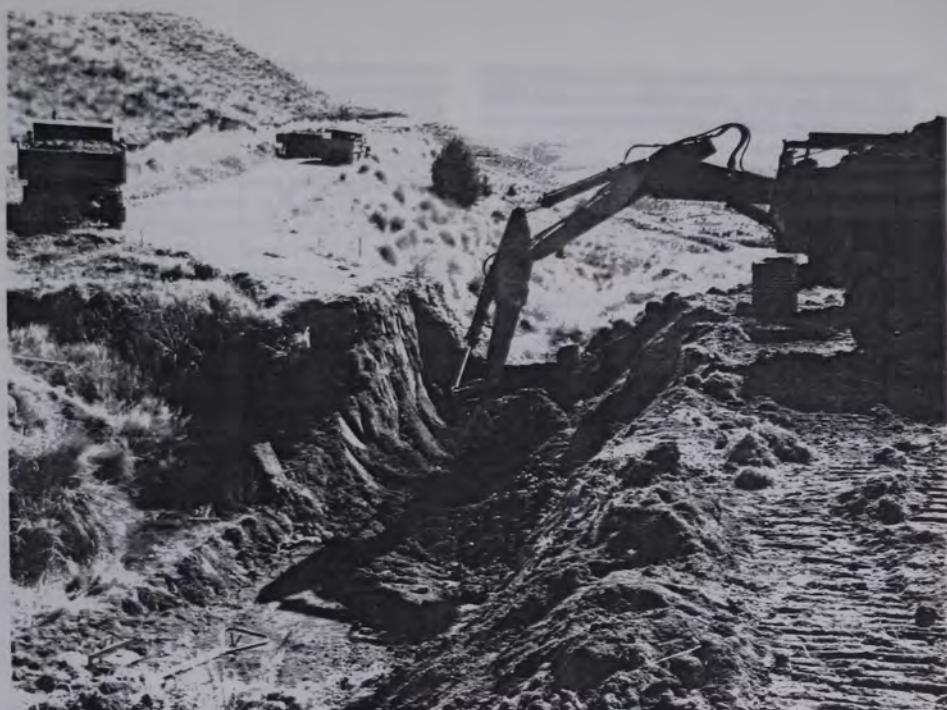
Excavating a trench for a culvert on the Imjin Road.
