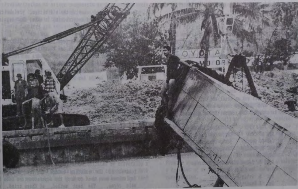
Barge at Harbour awaiting 'Righting' by heavy plant. Lt Hill aboard awaiting for lifting tackle.
