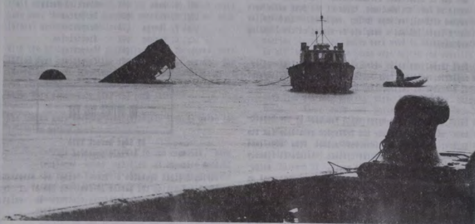
The newly raised barge being towed into Avatiu Harbour. (Notice air still being pumped in to avoid water coming into the holes and splits in the metal skin).
