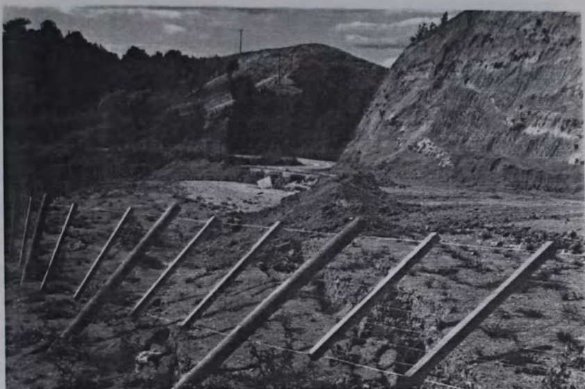
Above. Waingake Rd showing some of the damage. Notice the large cracks in the foreground and the dropout in the middle of the picture.
