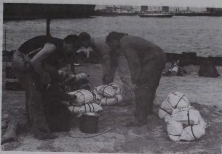
Photo 2 Preparation of 10kg charges
