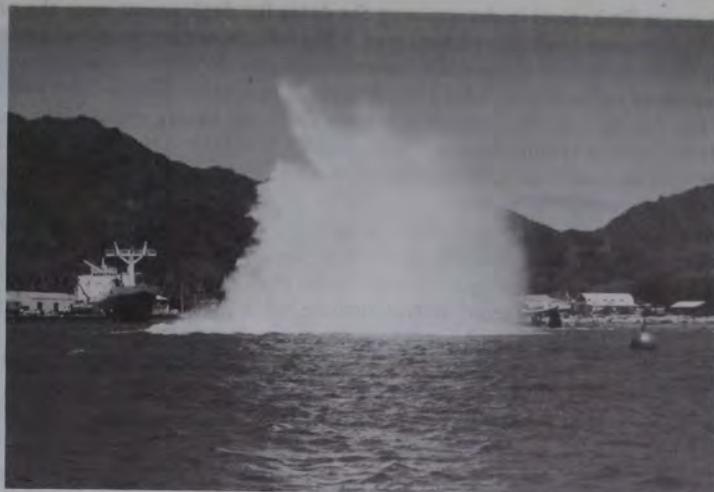
Photo 1 Coral blasting on Rarotonga. A 30kg ringmain is initiated.
