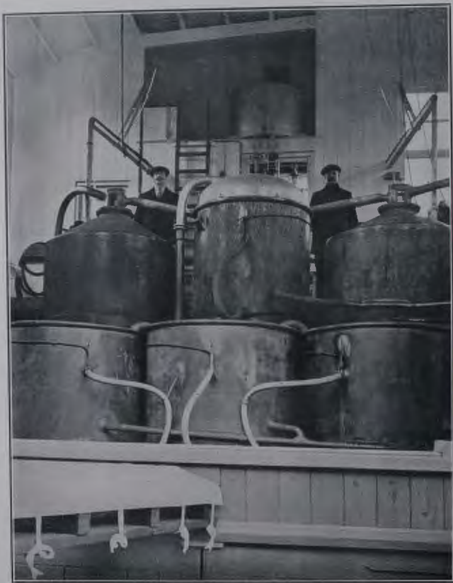
FIG. 11.3.—Interior of Nitrator House, showing Nitrator-Separator.
