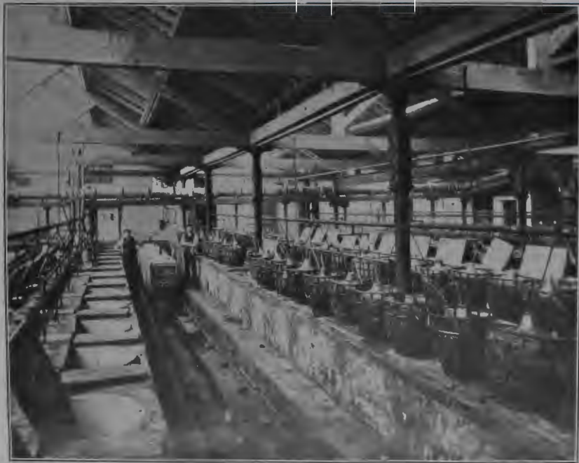
FIG. 6.2.—Picric Acid Manufacture. Pot Process.
