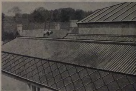
Photograph showing Asbestos Tiles and Corrugated Iron after covering by TURNERISED PROCESS. Note original appearance is retained.
