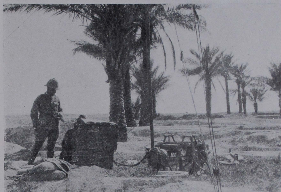
C Station with the Cavalry, erected during the operations on the DIAL and Khalis Canal. Note the arrangement of apparatus, also reels on which the aerial wire was wound. The officer is Captain Hillary.
