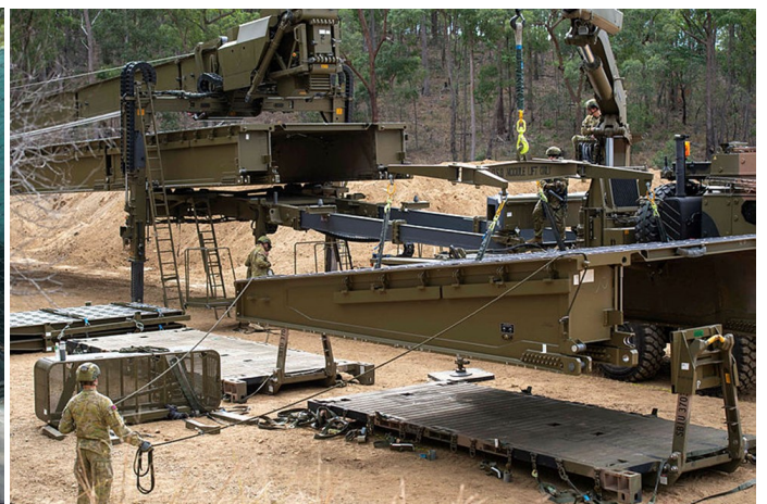
Figure 2: Construction of a Dry Support Bridge (DSB) during the Regiment's refresher training at Gallipoli Barracks, Brisbane.
