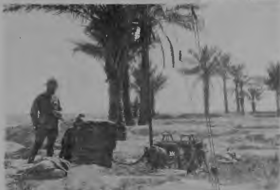
C Station with the Cavalry, erected during the operations on the Diala and Khalis Canal. Note the arrangement of apparatus, also reels on which the aerial wire was wound. The officer is Captain Hillary.
