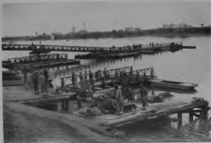
Indian and British Engineers of the Eighth Army spanning the River Po with a 1,370 feet pontoon bridge, the longest military bridge in Italy
