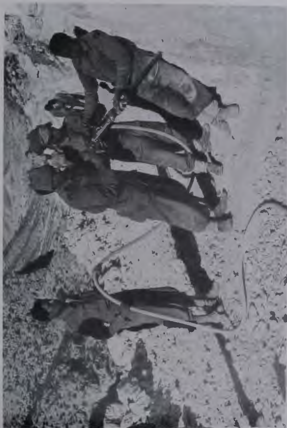
Using a pneumatic drill while roadmaking in Tunisia
