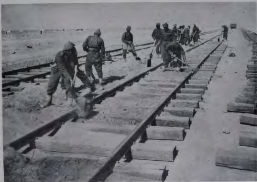
Indian Engineers laying railway track in Iraq
