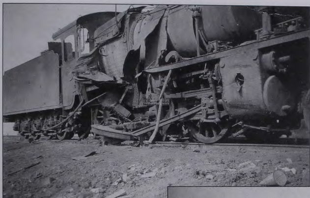
Above: One engine we left behind. A demolition charge was put in the fire box to render it useless to the Germans (E.S.R. 590).
