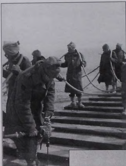
Left: Drilling holes for the dogs which fastened the rail to the sleeper.
