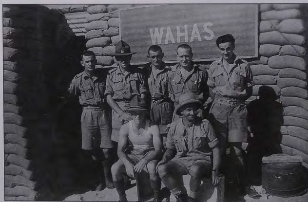
Earlier stations were built with corrugated iron; later the method changed to sandbags as added protection from aerial attacks.
