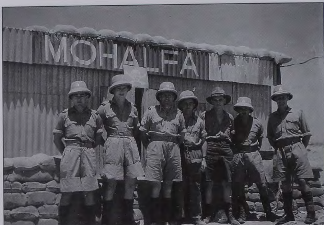
Earlier stations were built with corrugated iron; later the method changed to sandbags as added protection from aerial attacks.
