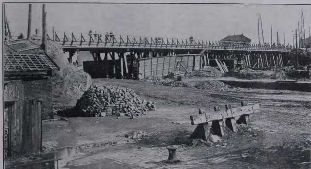
Photograph LI.—R.S.J. Bridge on Timber Trestles at Valenciennes, 350 ft. long.
