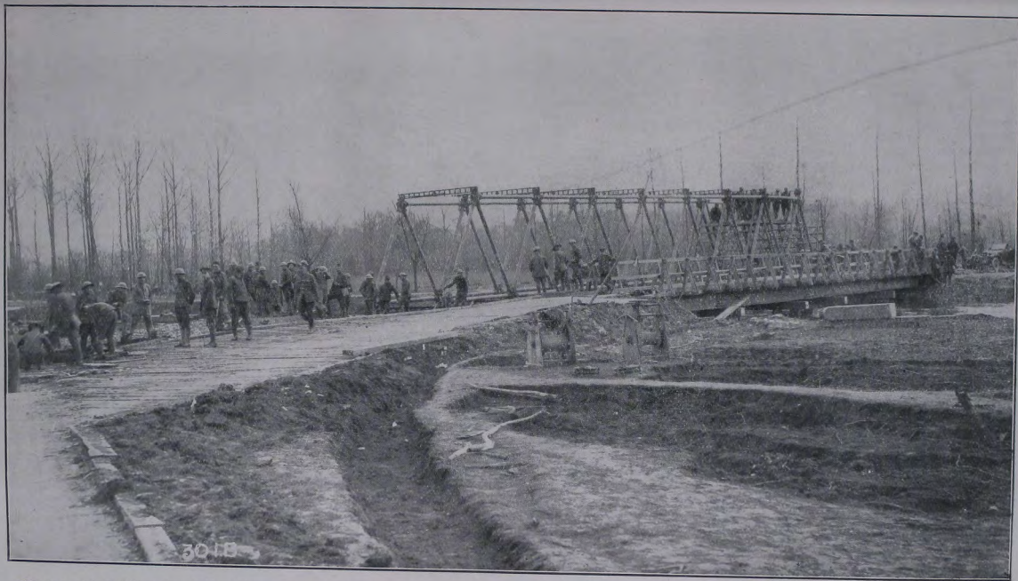
Photograph XXIV.—K. 84-ft. 0-in. length of Inglis Rectangular Type at La Motte, April, 1918; also to the right is shown K1, Replacement Bridge, consisting of 2 21-ft. 6-in. and 2 16-ft. 0-in. Spans, Mark II. N.14.d.1.3. View shows Inglis Bridge being dismantled. 4th Army.
