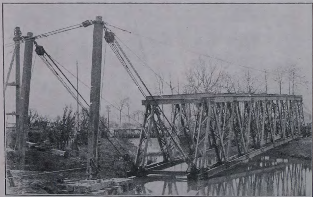
Photograph IV.—Launching Hopkins 120-Ft. Type Span. Span launched 100 ft.
