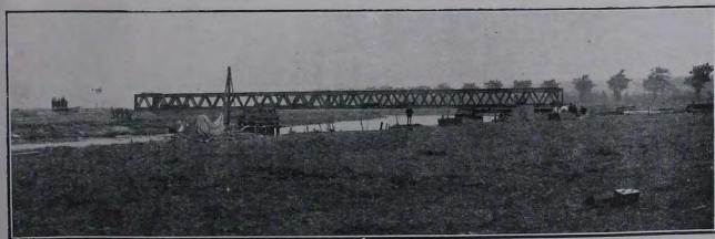
Photograph XX.—Erection of a Two-Span 85ft. Bridge at Beutin.
