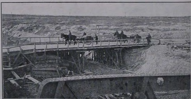
Photograph XXXII.—Canal du Nord : R.S.J. Spans for all loads.
