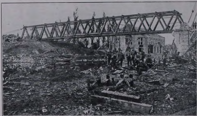
Photograph XXXVII.—Construction of 150-ft. Hopkins Bridge, Pont de Nieppe.
