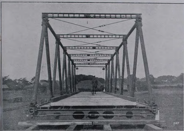
Photograph XV.—Inglis Bridge: Strengthened Type.
