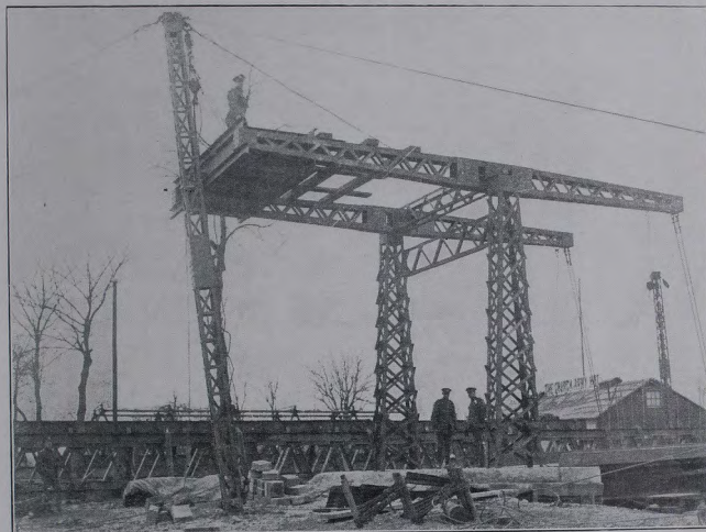
Photograph IX.—Pont Levis. Showing derrick used in erection.
