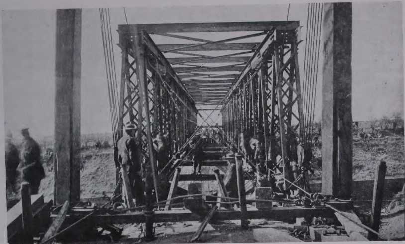
HAVRINCOURT BRIDGE. LAUNCHING JUST COMPLETED.
