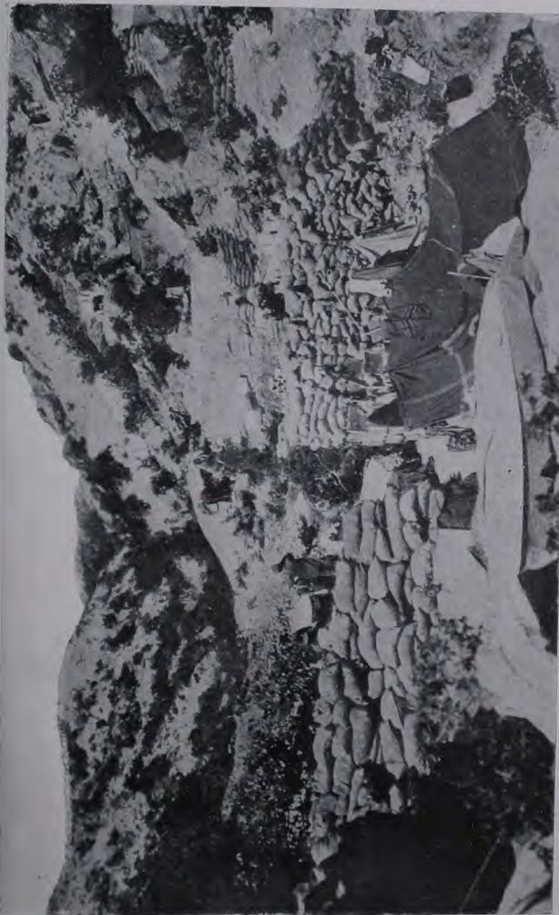
As the Turkish snipers at the head of Monash Gully could enfilade stretches of the road, sandbag traverses were built at the most dangerous points. [Lent by Sergt. P. Tite, N.Z.E.]
