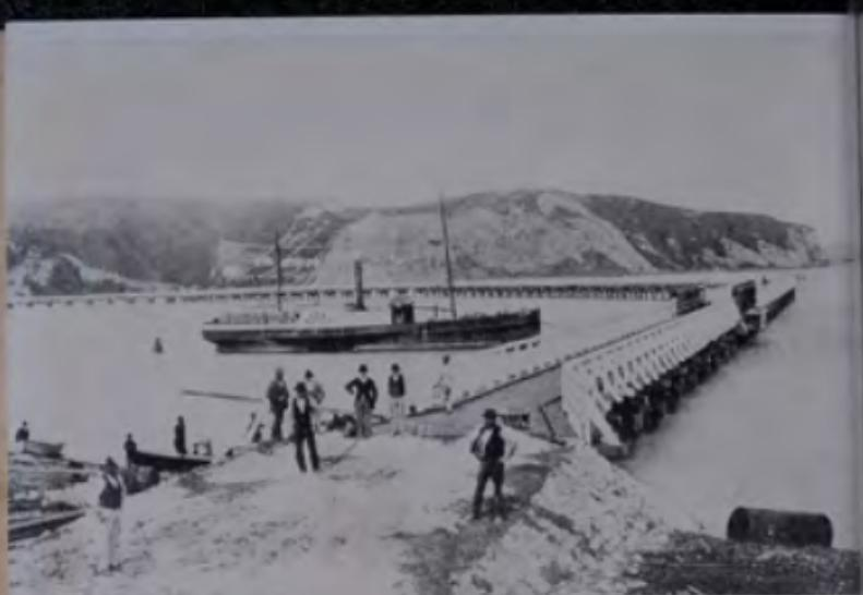
Westshore road bridge, Napier, designed by E. H. Bold, and opened in 1884. It had opening spans at each end. The paddle steamer is the *Mataia* which ran between Napier and Wairoa.
