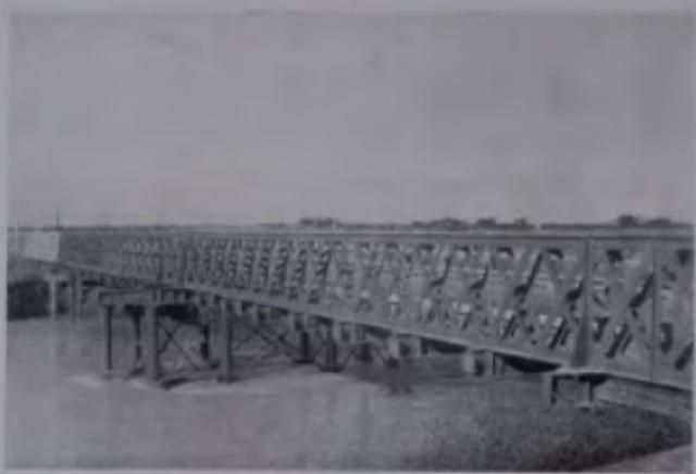
The Oreki iron bridge was built in 1865 and is still in use. It is founded on screw piles and was fabricated in Scotland. Originally, it is said, for use in the Crimean War.
