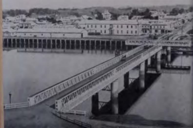
Wangamui town bridge with swing span open. The bridge was erected in 1869 by Kennard Bros., contractors, London. W. H. Hales was in charge for the Government. The bridge is still in use.
