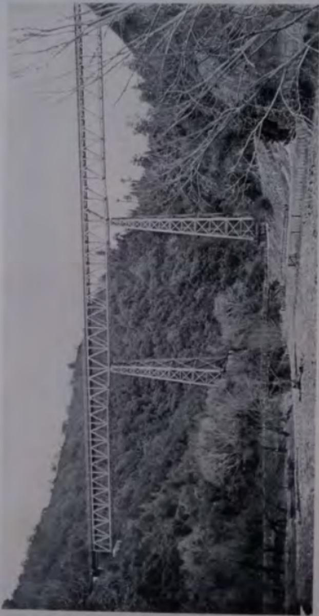
Makohine Viaduct on the North Island Main Trunk Railway, was designed by P. S. Hay and fabricated and erected by the Public Works Department. It was opened for traffic in 1902. It is another good example of the early local design and construction of a major engineering structure, and with some later strengthening has carried the Main Trunk Railway traffic for over 50 years.
