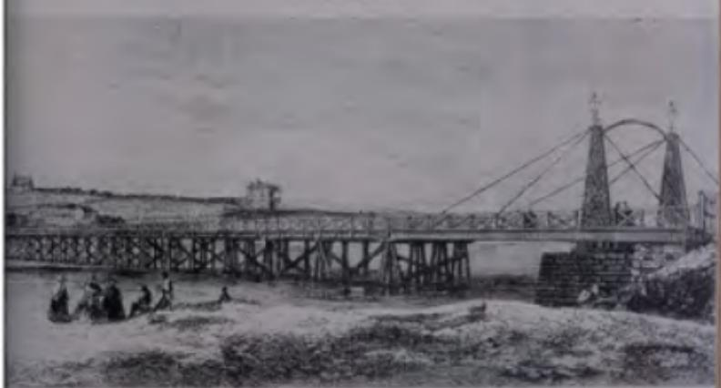
Tamaki bridge at Panmure, is one of Auckland's earliest bridges. It was built by the Provincial Government and completed in 1865. It was 576 feet long, with a 21 foot roadway and an opening span giving a 40-foot clear waterway for passing vessels. The opening span was not in use for long, but the bridge itself was not replaced until 1916.
