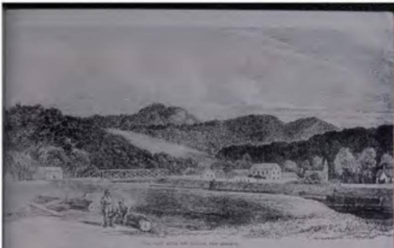
The first Hutt Road bridge, a single-span truss bridge, built in 1848. It was badly damaged during the earthquake of 1855 and completely destroyed by a flood shortly afterwards. The site was near the original Fort Richmond on one side of the river, and Mr. F. G. Molesworth's property on the other.
