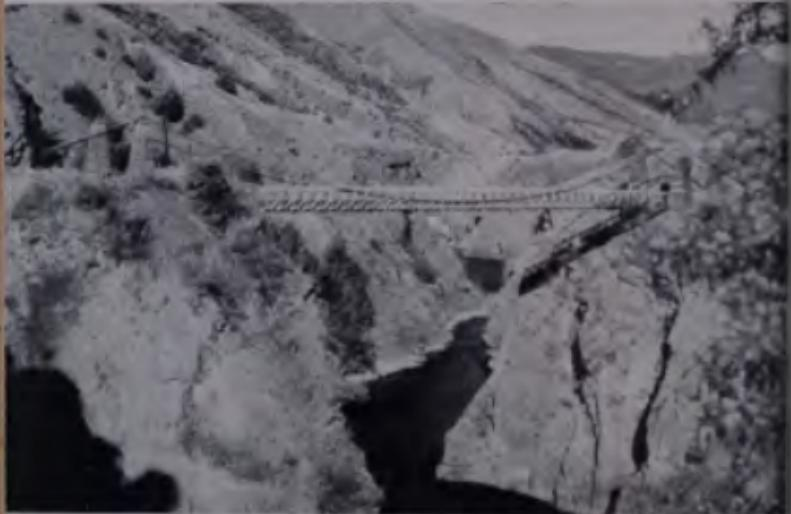
Kawarau River suspension bridge, designed and constructed by H. P. Higginson. It was opened for traffic in 1880, and after 73 years is still carrying heavy modern highway traffic. The span is 300 feet.
