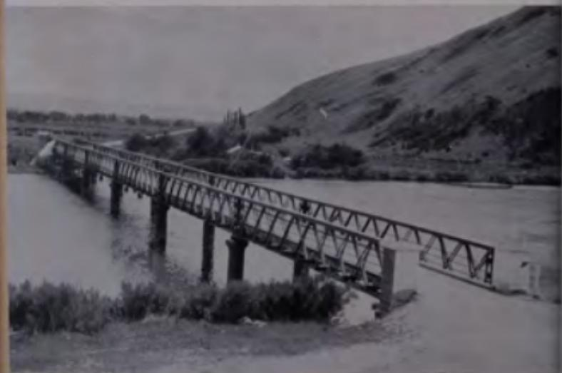
Taieri River road bridge, Henley, erected during 1883-84, replaced one erected in 1863. It is constructed of six wrought iron trusses of 80 feet span, carried on cylinders, and is still in use.
