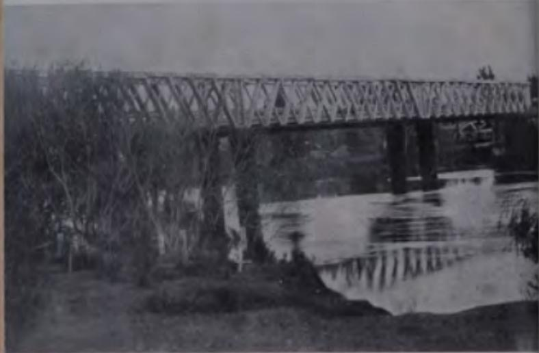
Waikato River railway bridge at Ngaruawahia was built about 1876 and with some strengthening carried the Main Trunk Railway traffic for 55 years. It is still in use as a road bridge.
