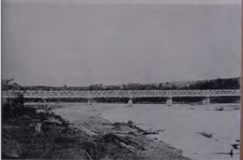
Rangitikei River road bridge at Bulls. The earliest bridge in the Manawatu area, it was built during 1873-74, but was carried away by the flood of 1897. It was of six spans of about 80 feet each.
