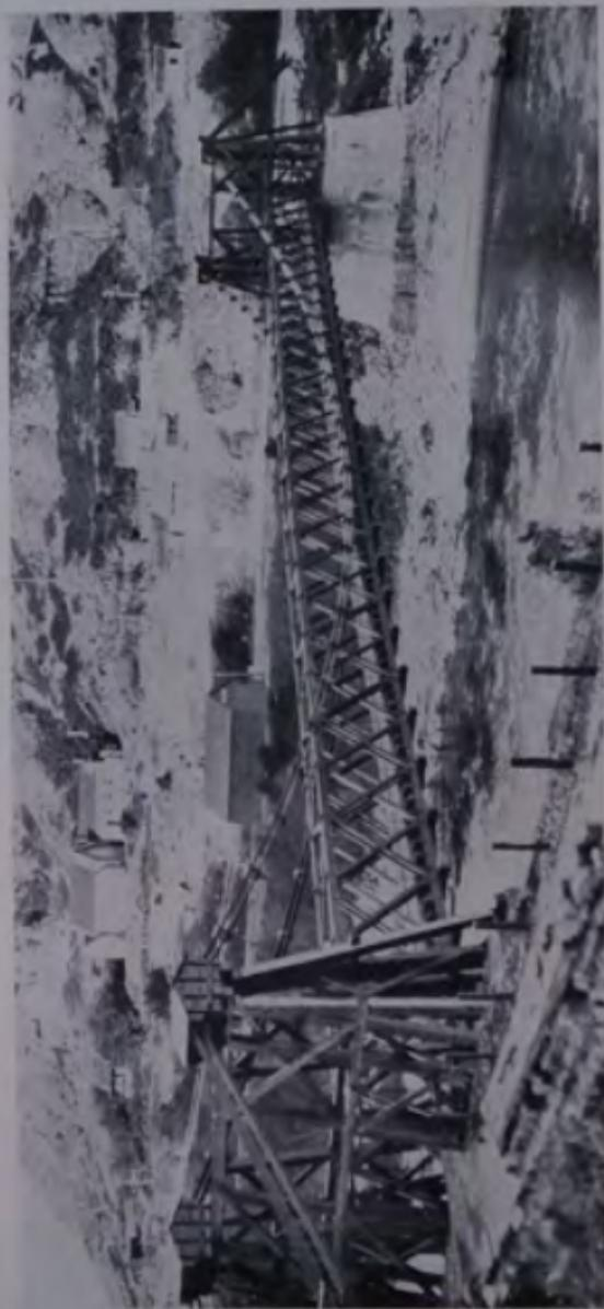
Britannia suspension bridge. The first bridge of similar design collapsed in 1876 just as it was completed. Failure of the main anchor plates was apparently the cause. The span is 300 feet.
