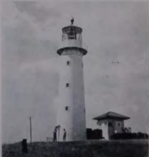
Tiritiri Lighthouse, the second built in New Zealand. It is of cast iron fabricated in England. It was first lighted in January, 1865, and is still in use with modern illumination.
