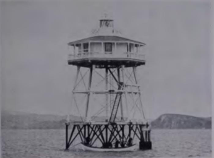
Ponui Passage Lighthouse, built during 1870-71, was founded on screw piles originally intended for the Wellington Patent Slip. The substructure is still used to carry the new light.
