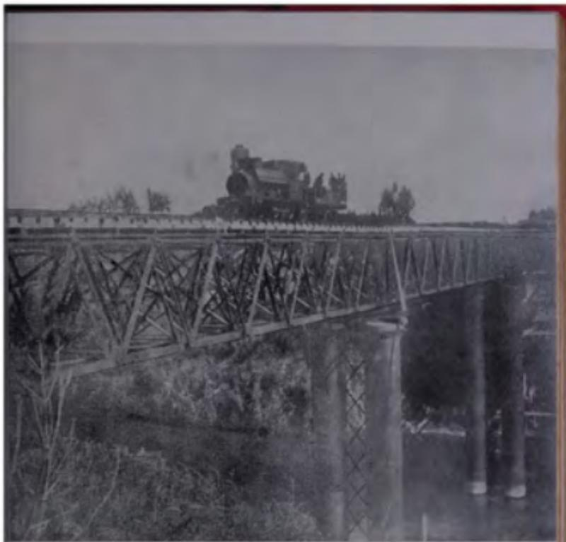
Waikato River railway bridge at Hamilton. Completed in 1883. A good example of bold design of an early railway bridge. The main spans are 132 feet supported on cylinder piers and the rail level is 99 feet above the river. The bridge has been strengthened and is still carrying the heaviest railway traffic.
