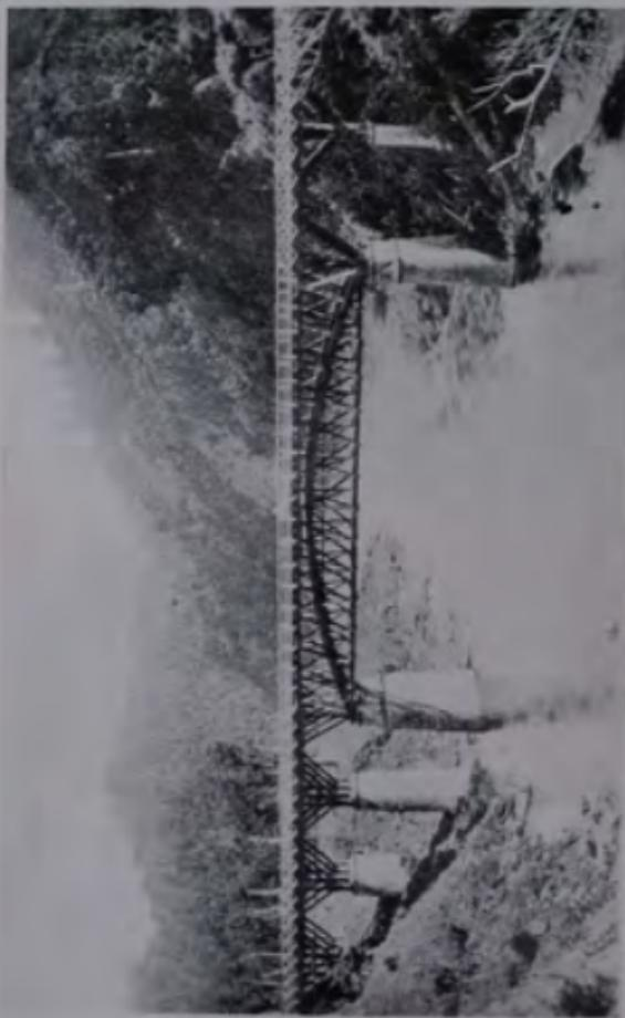
The Manawatu Gorge bridge was officially opened in 1875. The main span is 162 feet and the stone piers are 52 feet high. The timber was totara which was still in excellent condition when the bridge was replaced by a reinforced concrete structure in 1931. It was a toll bridge from 1875 until 1907.
