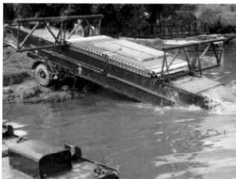
Class 30 Light Assault Floating Bridge. Pontoon being launched
