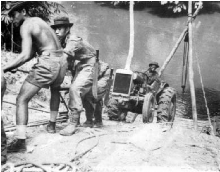
Fort Dixon Airstrip. A Ferguson tractor brought by boats in pieces and reassembled being hauled up the river bank by Malayan Sappers
