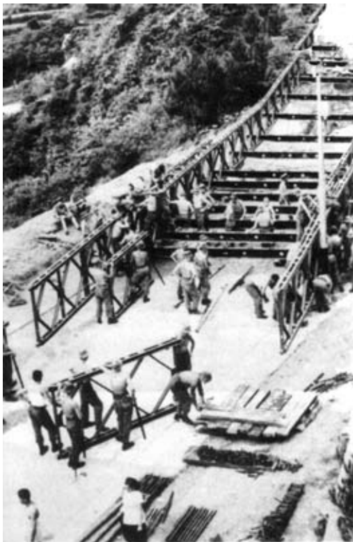
Bailey bridge under construction by 24 Field Engineer Regiment at milestone 3\frac{1}{2} on the Tai Po Road, Hong Kong, after a wash-out in 1956
