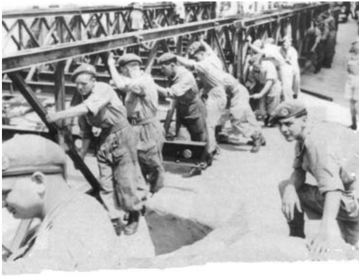
A Bailey bridge being built in Trieste shortly after the war to assist the civil population
