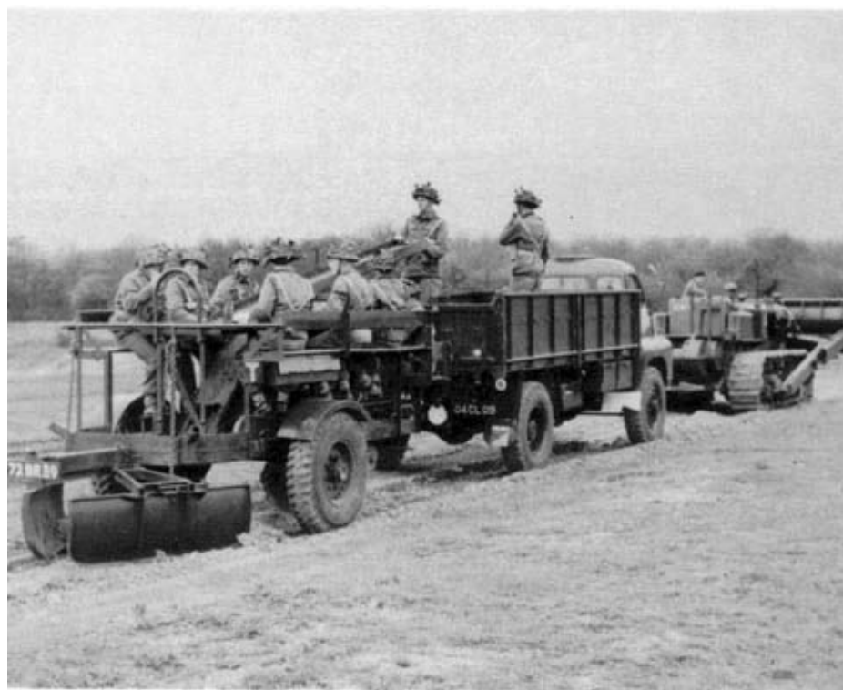
Minelaying train in action, laying Mk VII antitank mines (Courtesy of the Trustees of the Imperial War Museum)
