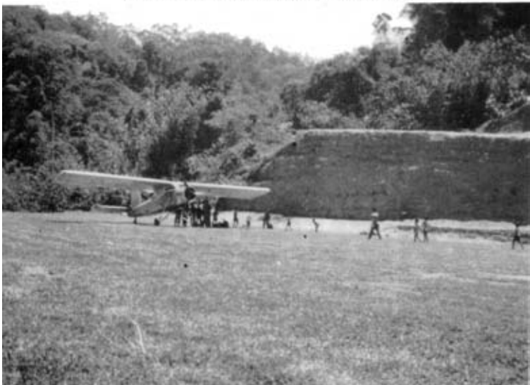
Fort Chabai airstrip. This view gives an idea of the very heavy earthwork carried out in some cases by light tractors imported by helicopter or boat
