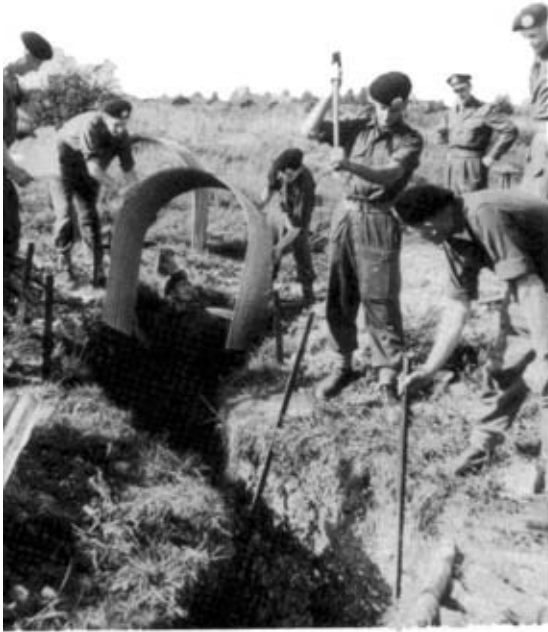
RE Officer cadets undergoing fieldworks training using hairpin shelters designed for protection in nuclear conditions
