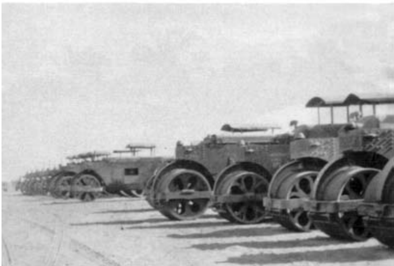
Tar boilers and road rollers at the plant depot, Quassassin, Canal Zone
