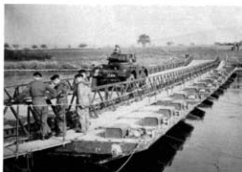
Class 30 Light Assault Floating Bridge complete, Hameln 1953
