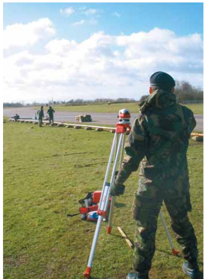
Figure 5 – Gravity fed drainage is given the correct slope.
