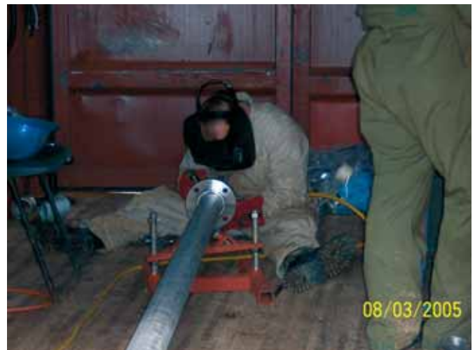
Welding a flange on the 3 inch stainless steel pipe
