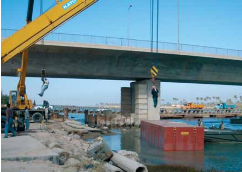
Pontoons being launched. Note the effective use of the crane hooks to retrieve the slingers from the launched pontoon.
