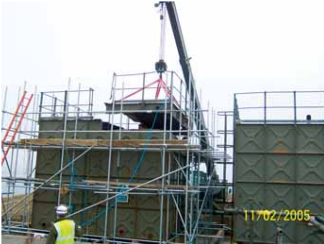
Braithwaite Aviation Turbine Fuel tanks being demolished.
