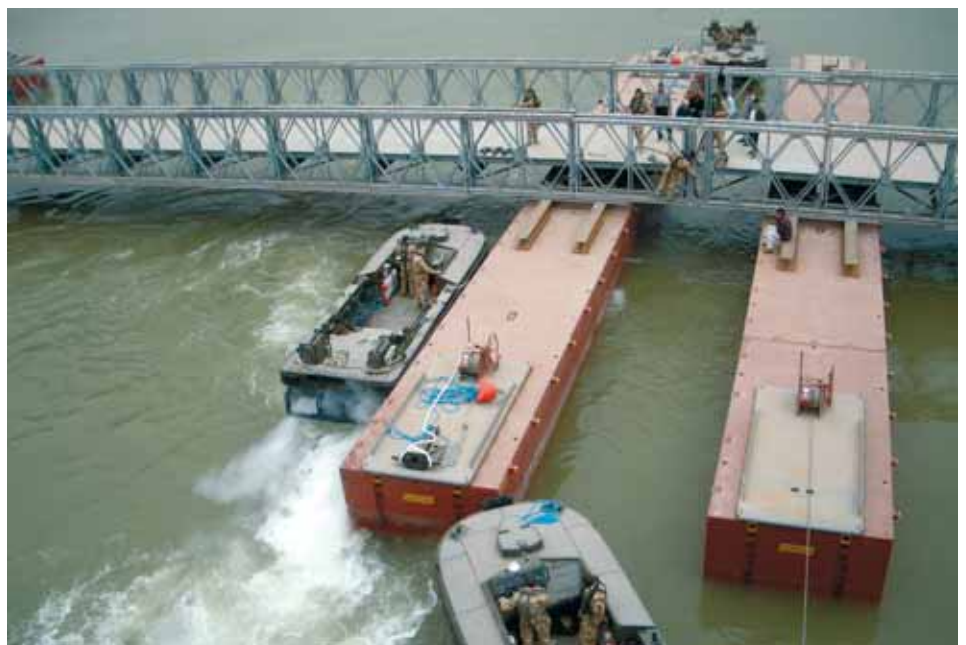
Applying pressure to join the bridge. Note the anchor has been deployed on the right hand pier, the left hand anchor is on the pier awaiting deployment.
