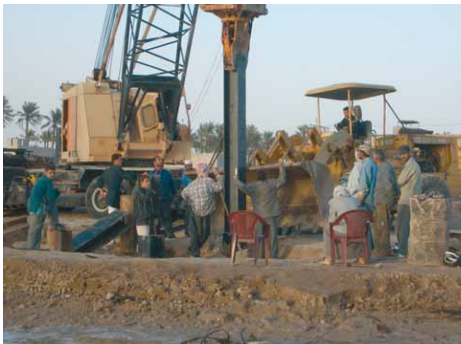
Pile driving on the earth causeway to form the H-pile causeway. Note the chairs for the supervisors!
