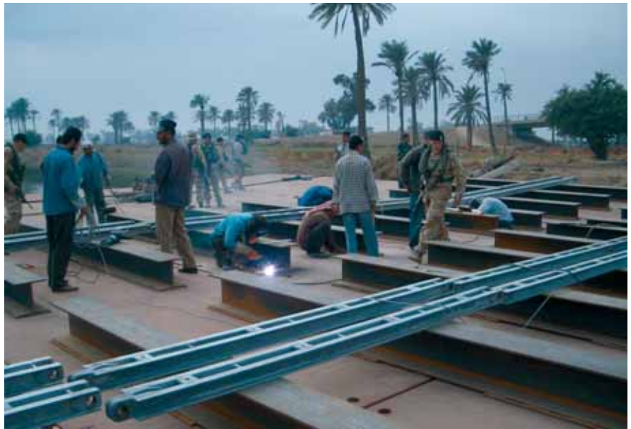
Welding the distribution beams on the floating piers. The reinforcement chords are then bolted to the distribution beams. The bridge panels connect to the chords.
