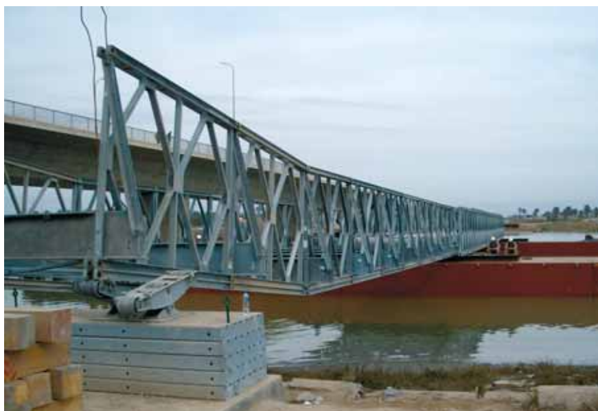
The back end of the span has landed on the inside floating pier and the articulated section of the tail is on the verge of running off the inside rollers.
