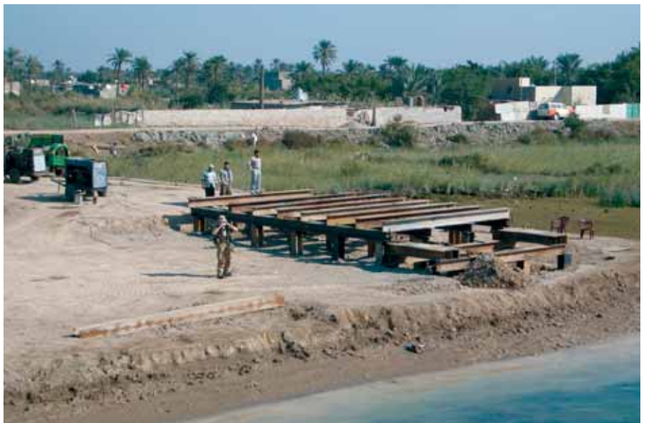
The H-Pile causeway (less deck) on the new “beach”. The original river bank can be seen in the background.
