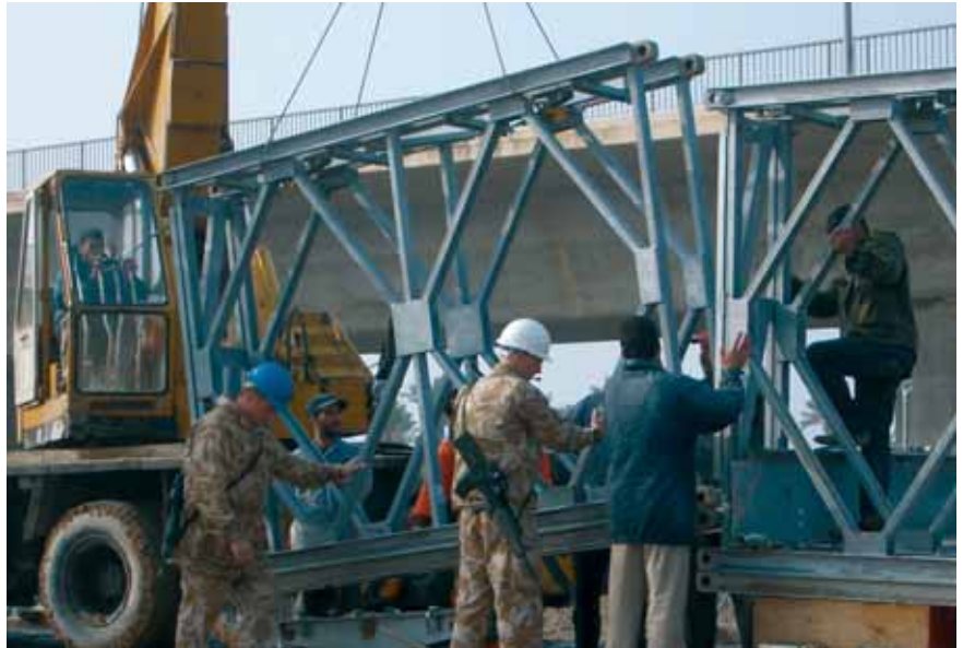
A double truss box section being fitted.
