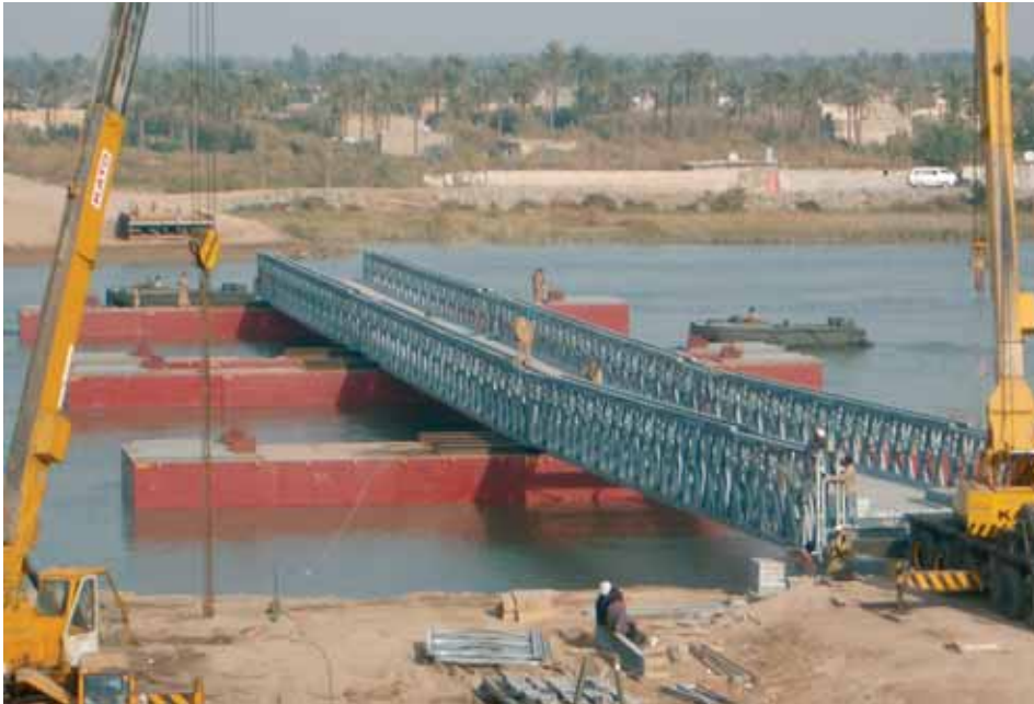
The home bank landing span and 2 floating spans complete.
