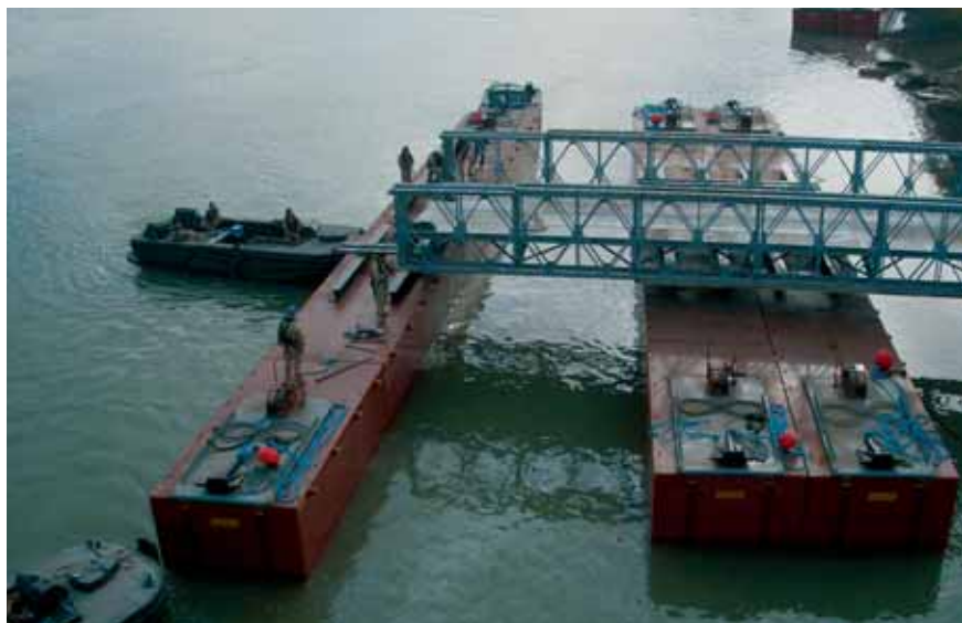
The end of the span is connected to the outside pier before the back of the span is landed on the inside pier.
