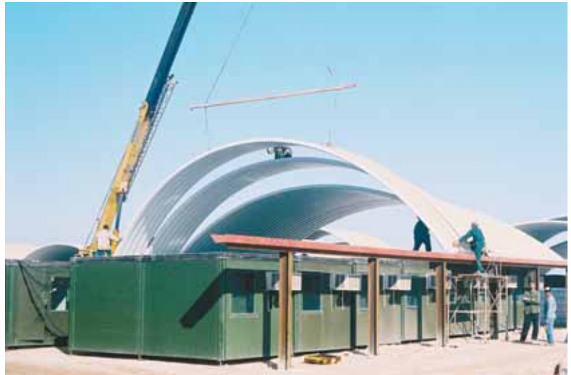
Figure 5 – Temporary Field Accommodation units being over-roofed.
