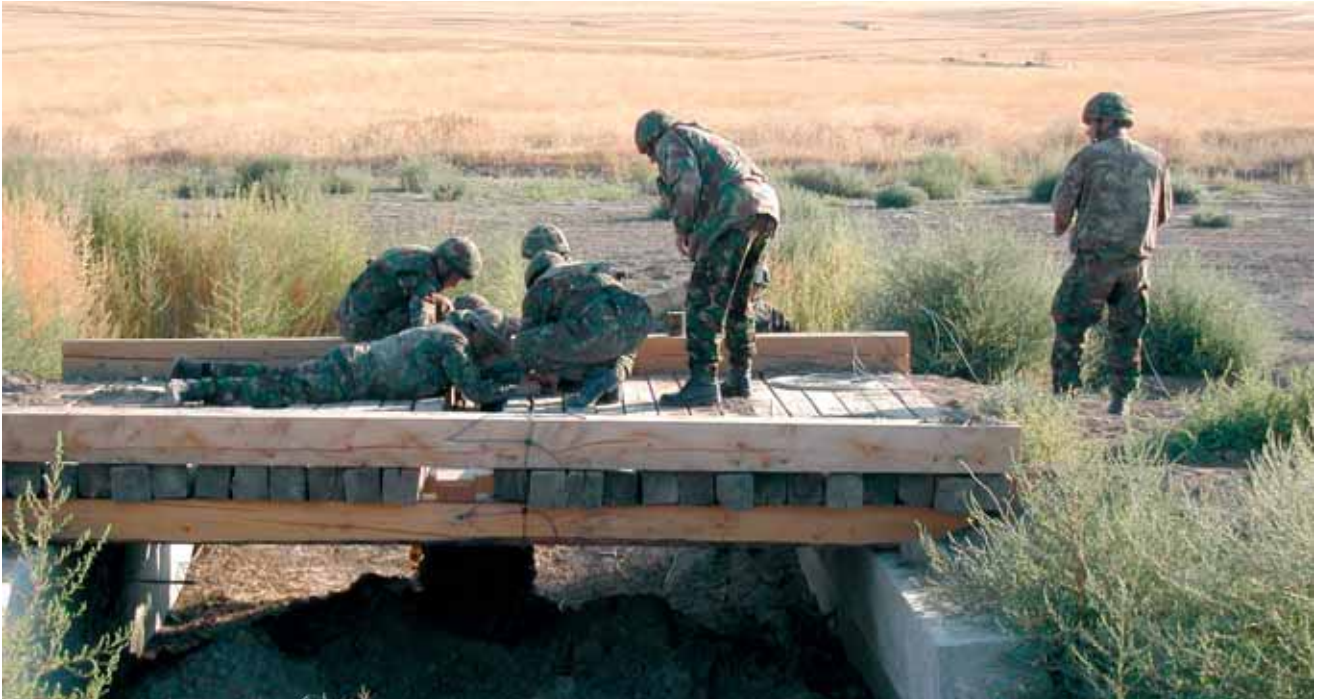
Preparation of an NEB for demolition during the live firing phase of Ex Iron Anvil 03.
