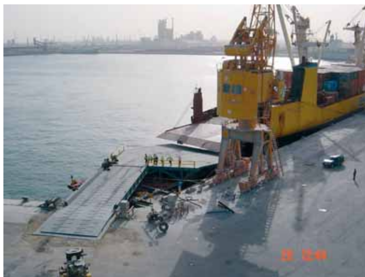
Kuwait Docks did not enable Ro-Ro unloading at a full tidal range and so, with Engineer and Logistic Staff Corps advice, a contract was let for a Ro-Ro platform.
