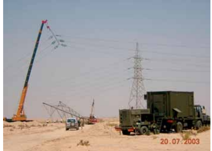
Helping restore the power infrastructure, in this case repairs to a 400KV Power Line.
