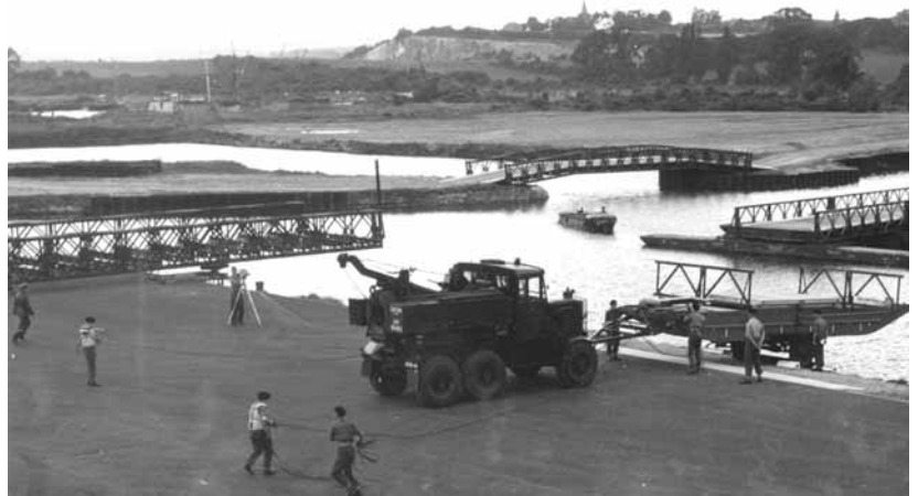
A Scammel Heavy Recovery Vehicle launching the next bay.
