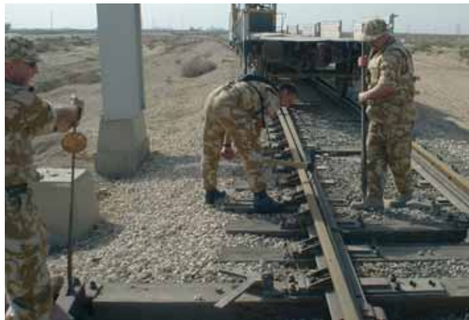
Repairing points north of Umm Qasr.
