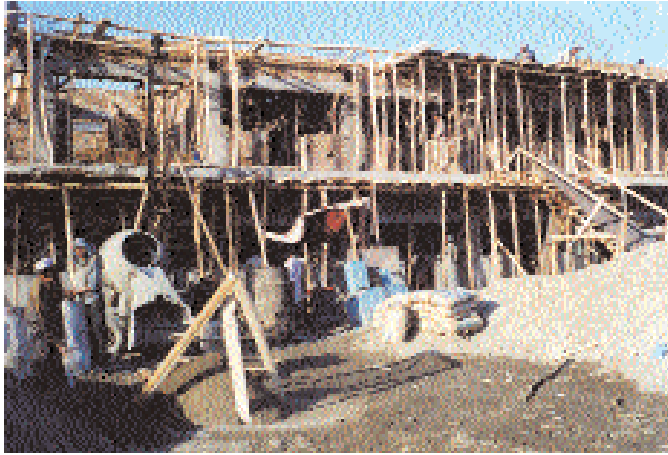
Accommodation Blocks: concrete batching plant and temporary timber supports.
