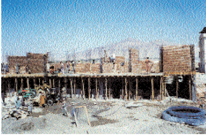
Accommodation Block: first floor slab with brickwork partitions and rebar to reinforced concrete columns.
