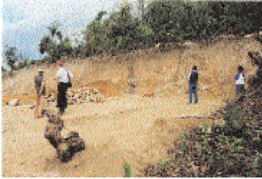
Over 3,000 cubic metres were excavated by hand at Thulowara to provide a site for the new High School.
