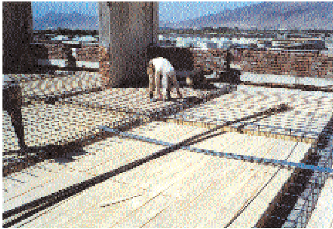
Exhibition Hall: first floor soffit for concrete slab in position with rebar being placed.
