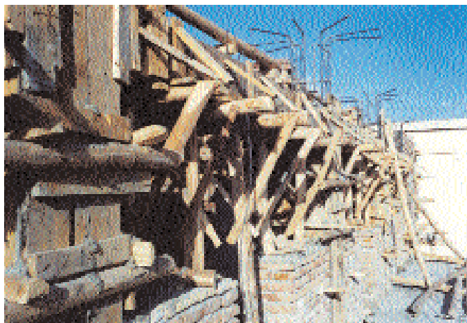
Accommodation Blocks: formwork to columns and edge shuttering to first floor slab.
