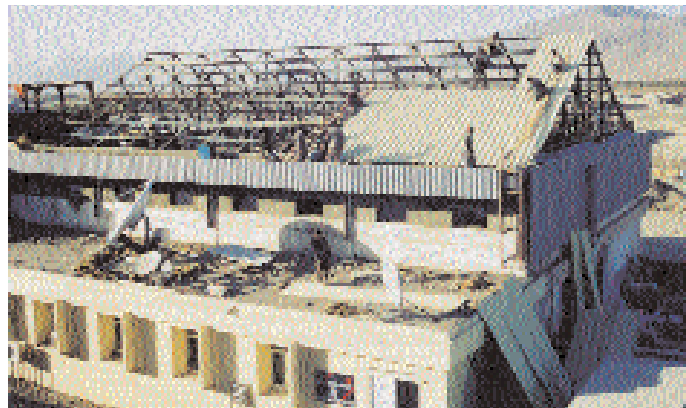
Exhibition Hall: Roof trusses in place and being clad with steel profile sheeting
