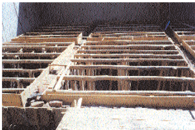
Exhibition Hall: soffit supports. First floor roof slab.
