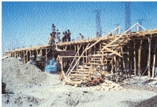
Accommodation Block: temporary stairway to first floor.
