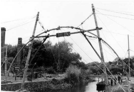
The first two ribs as constructed using 18th century techniques, prior to joining.
