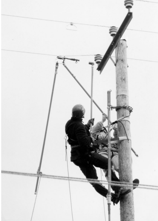
Pole Top Team securing a "Wedge Tap Bail"
