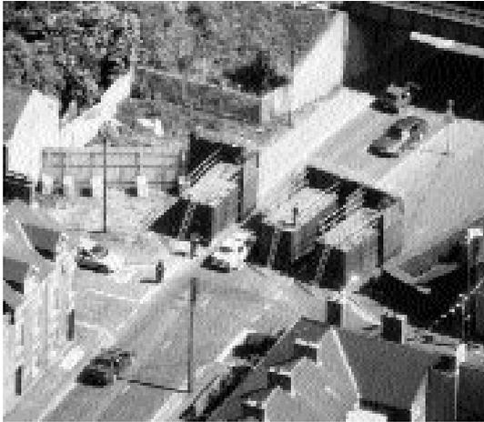
CCOs at Garvagh Road, Portadown. Doors open for vehicle and pedestrian access.
