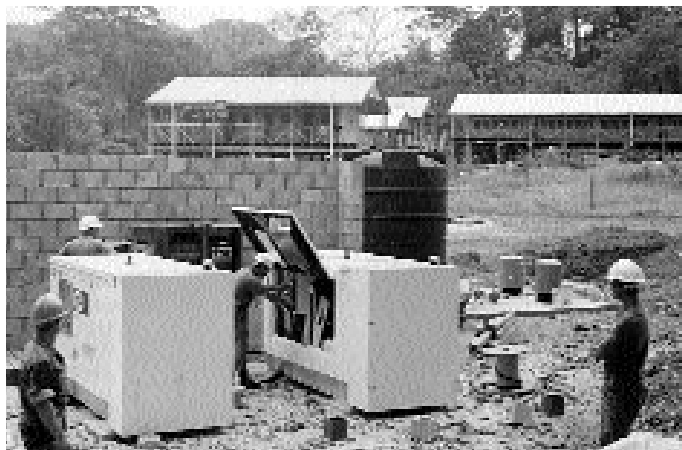
Installing the power generation and distribution system at La Sierra.
