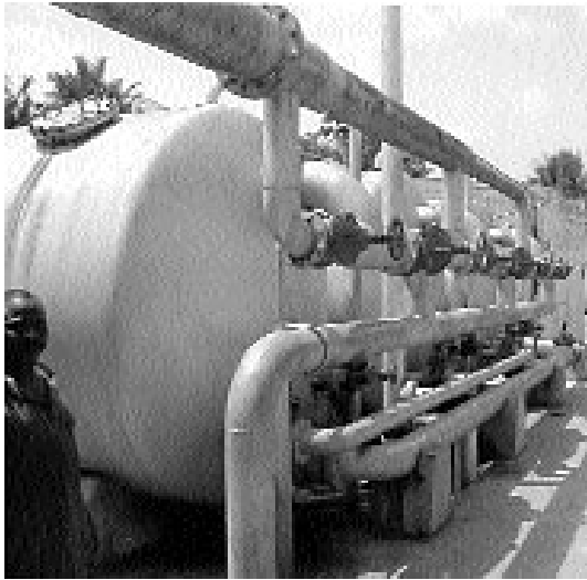
Water filters at the Sanda Water Treatment Works.
