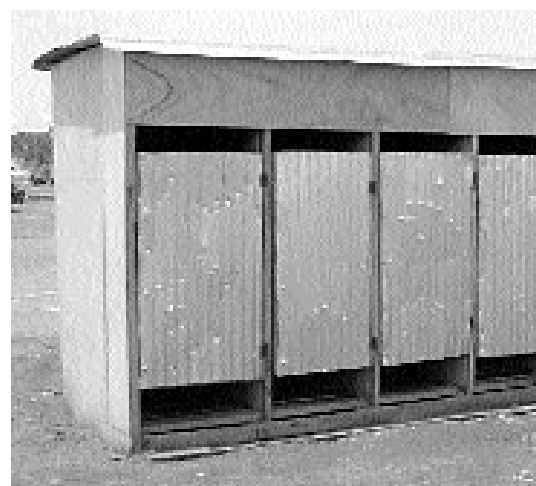
Pedestal deep trench latrine constructed of plywood when corrugated iron sheeting was in short supply.
