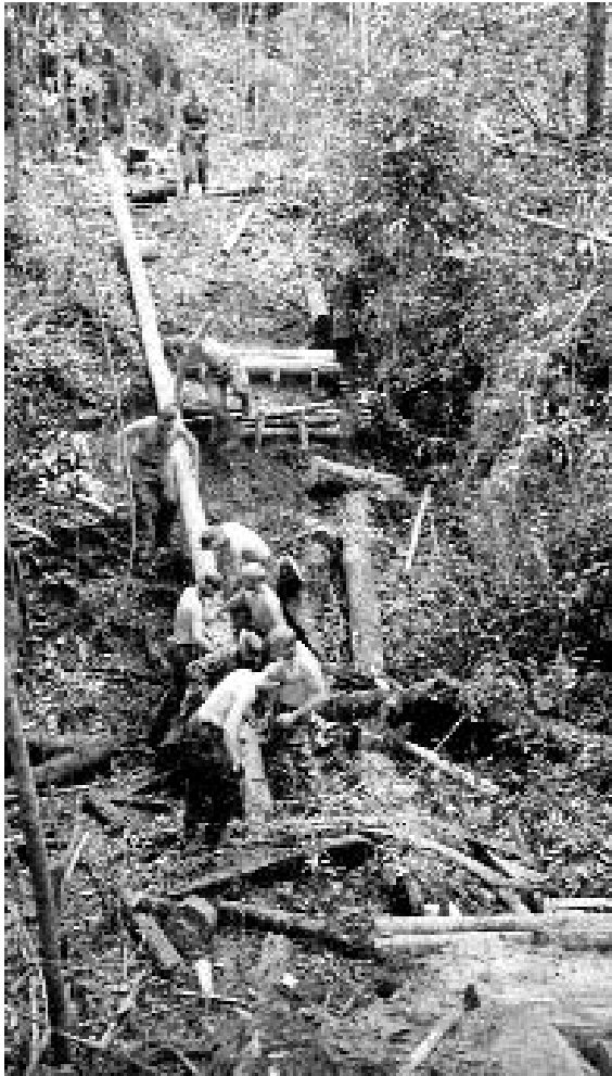
Zulu bridge, a 10m long non equipment bridge, is being constructed together with steps.
