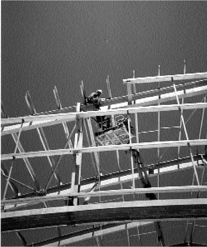
Tightening bolts at a height of 15m.
