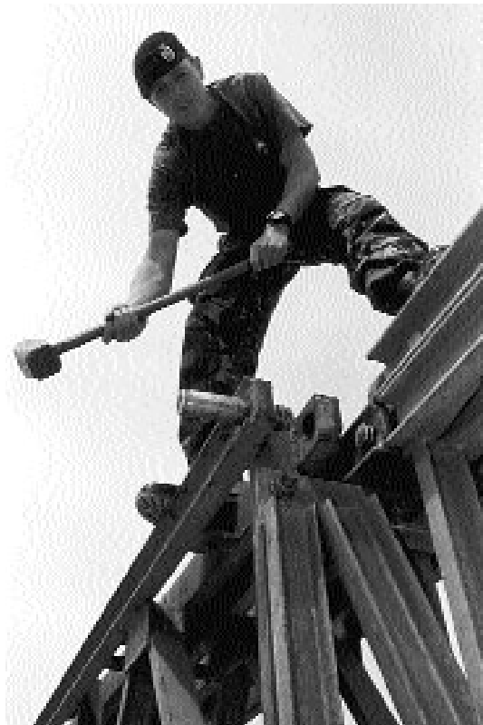
In-theatre logistic bridging; critical to the Army supply chain.
