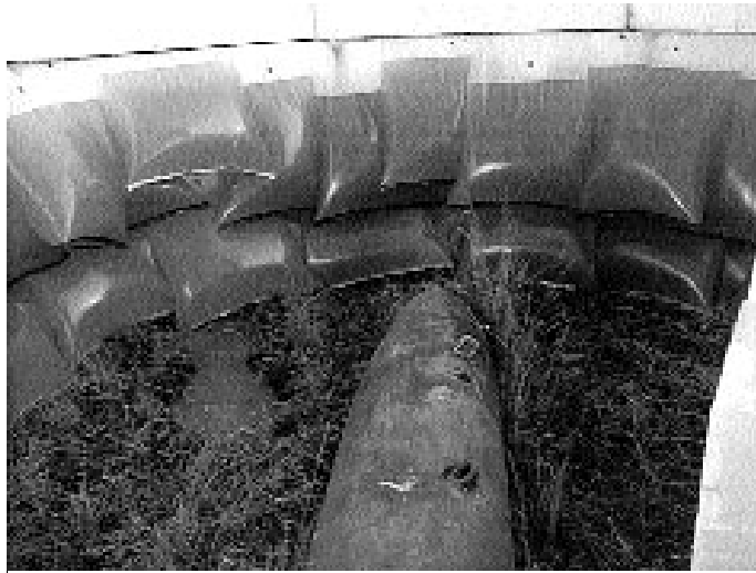
Water suppression equipment constructed around an unexploded Mk 84 2000lb bomb.
