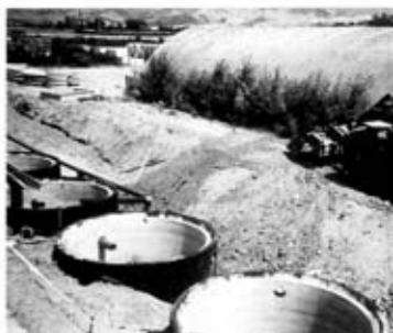
Backfilling.
