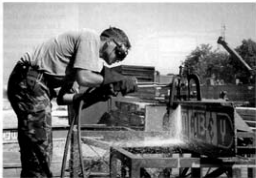
Sapper Wilson adapting bridge components.
