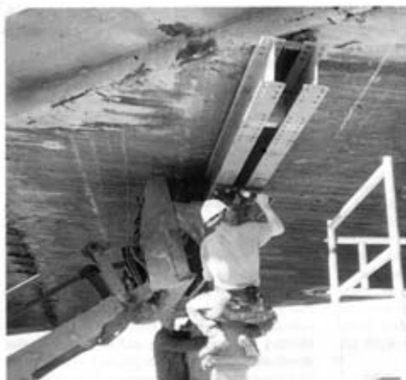
The bridge seat beam, held in the jaws of a light wheeled tractor bucket, is bolted onto the jacks.
