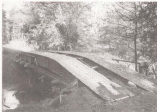
A No 10 close support bridge used to overbridge a dodgy wooden structure in Poland. Note the 1m gap: a serious problem for CVR(T), Land Rovers and B vehicles.
