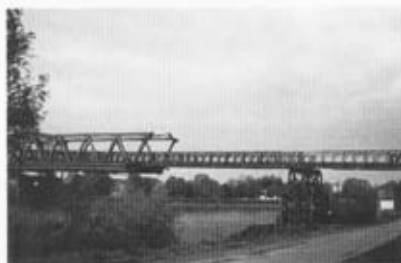
The completed bridge at Stara Gradiska. Note the position of the end of bridge over the existing bridge pier.
