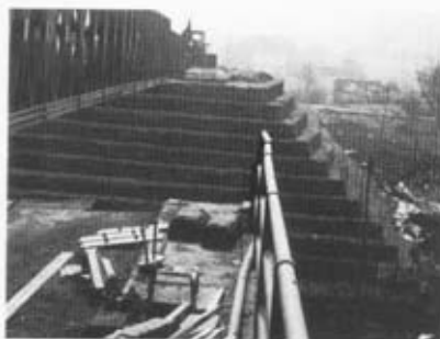
The 21-bay triple single reinforced bridge at Visoko just before launch – note the wire gabion pyramid on the far bank.
