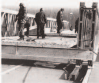
The end of the bridge at Brcko – note "I" beams on inner panel line and outer line resting on the kerb.
