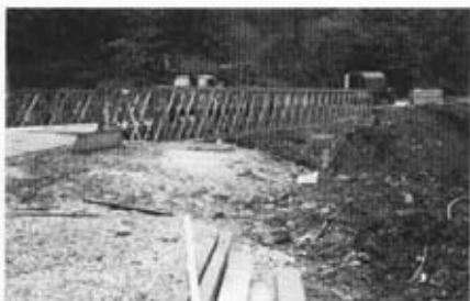
The completed bridge on Route Python. The photograph has been taken along the direction of launch showing the distance the bridge had to be moved into its final position.
