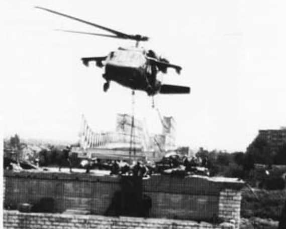
Support frame being positioned at central pier.
