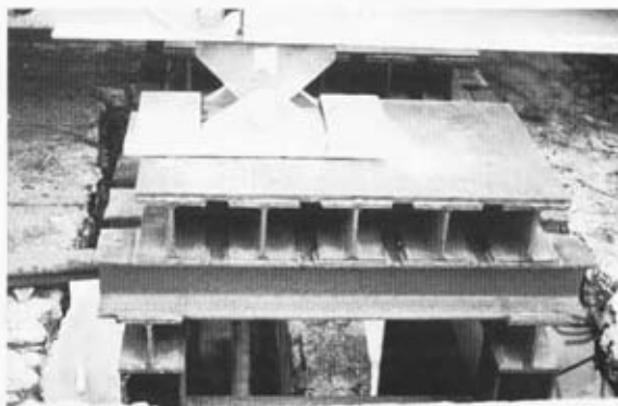
Support at Pier G. The base plate is in its final position, 220mm to the right of the pin above, its originally designed position. The additional UB is in position below the grillage. Web stiffeners to UB, directly above the supporting columns to be added.
