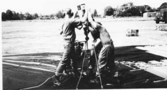
Use of a hydraulic hammer to fix retaining pins into hard clay.
