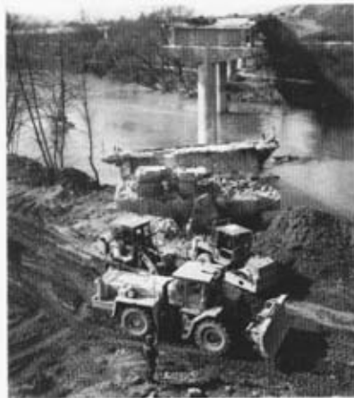
Preparation of the Visoko bridge site is carried out by German engineers before construction by German, Romanian and Austrian engineers and drivers, of a 55m Compact 200 bridge.
