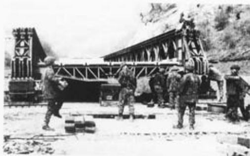
The Ross bridge grillage construction.
