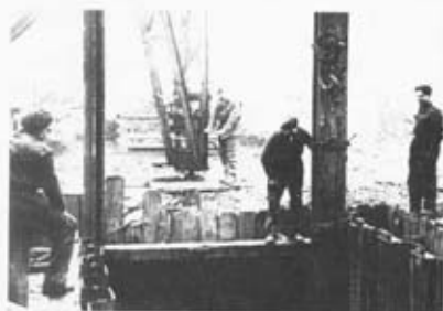
Sheet steel piling can be seen inside the timbered shaft.
