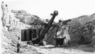
Figure 2. Quarrying of weak Middle Jurassic limestone near Carpiquet, August 1944, using a 30-ton shovel. The rock, known locally as Calcaire de Caen (cf. Fig. 7), is of Bathonian age and similar to the Bath Stone of the Cotswolds in southern England. It occurs as near-horizontal strata. (Copyright The Imperial War Museum, London; Photo CL811).
