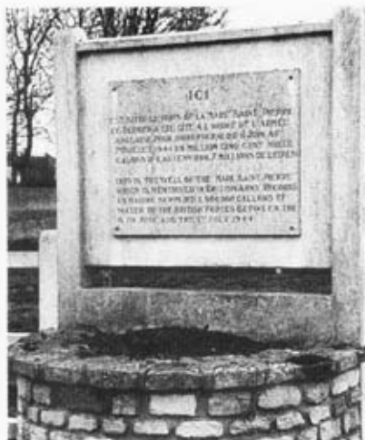
Figure 6. "Well" at Hermanville-sur-Mer. However, the apparent well-head is a postwar memorial. The water source was probably the local pond (mare), since the hydrogeological setting and calculated abstraction rate make a borehole source unlikely.
