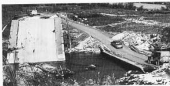
The site of the future Neames HGB bridge. Left: 61m gap on original alignment. Right: pontoon bridge (MLC 55 on a good day.)
