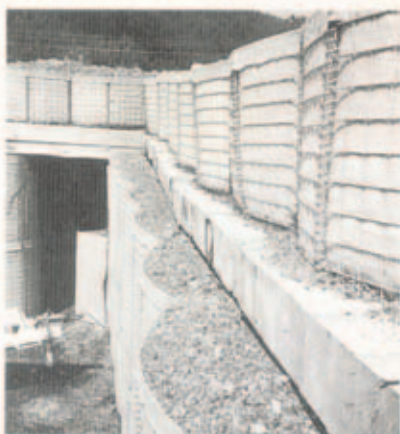
A standard design COLPRO. This Hesco-Bastion fill has settled due to poor compaction causing the roof to sink. Note the small gap between the fill and the roof timbers - there is a roof support beam that has sunk, between them.
