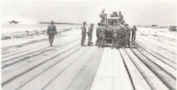
Figure 7. Sappers using a "stampclicker" to pave a temporary airfield in Normandy with Prefabricated Bituminized Surfacing (PBS). Developed by the Canadians from a British origin, PBS gave a better surface than SMT but was slower and in high winds more difficult to lay and was therefore less commonly used. (Copyright: The Imperial War Museum, London; Photo CL468)
