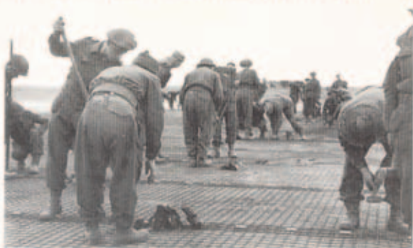
Figure 6. Sappers surfacing a temporary airfield in Normandy with Square Mesh Track (SMT). (Copyright: The Imperial War Museum, London; Photo CL468)
