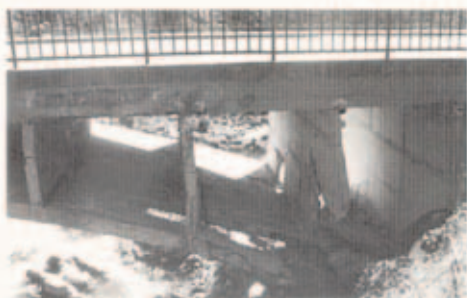
Side view of the bridge showing the damage to the three spandrels and arch. The original extent of the river below can be seen clearly.
