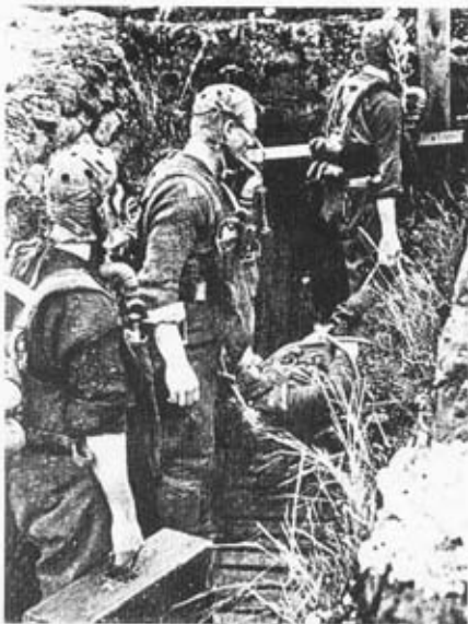
Proto men at Rex Smart's First Army Mine Rescue School, demonstrate a mine stretcher. Twin oxygen cylinders were carried at the rear and carbonate of soda on to the left of the chest. (Logan 1923)
