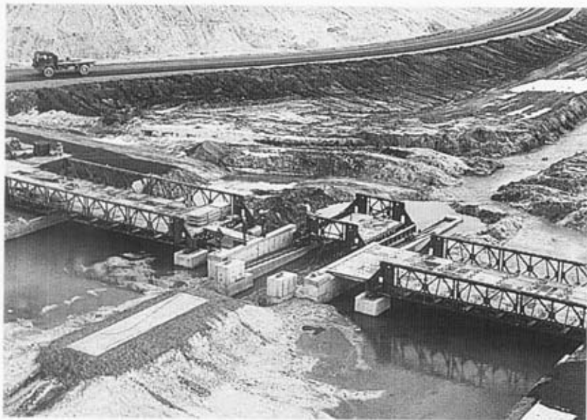
Photograph showing bridge gap 2 nearing completion with sliding span in open position.
