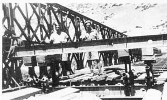
Aliakmon Bridge jacking arrangement.
