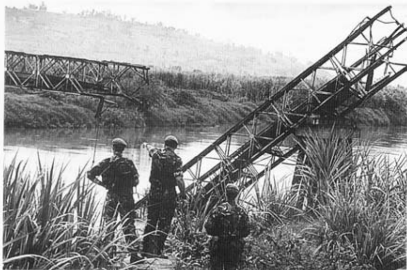
OC, 2IC and SSM 9 Para Sqn, viewing the damaged Kanzenze Bailey bridge, later reopened by the squadron as the longest bridge in the country.
