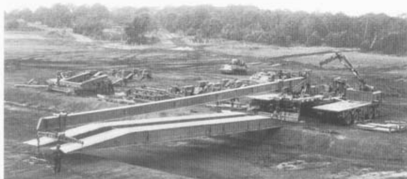
GSB vs MGB. 32m GSB almost complete after approximately 16 minutes. MGB still has some way to go!
