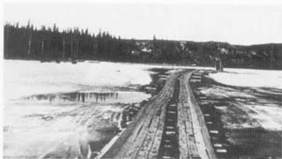
Plank and sawdust road across ice on Peace River, March 1942. Credit: Office of History, US Army Chief of Engineers.
