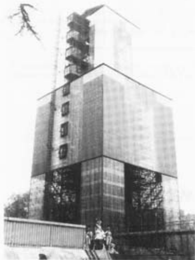
E/M of free-standing scaffolding encloses the Albert Memorial during essential repairs. Marble group representing "America" in the foreground.
