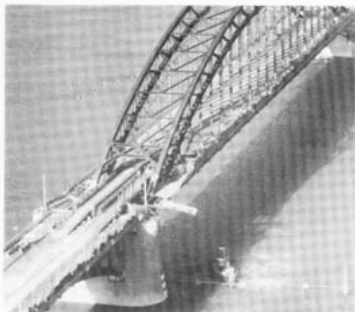
The Nijmegen road bridge showing the two 800 Double Single Bailey bridges over the gap caused by the enemy frogman. Crown copyright
