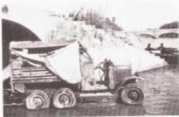
Second lorry after three days' immersion. (Note upstream "salvage raft" with its two winches just beyond steps.)
