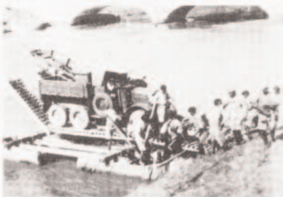
IMPROVED RAFT WITH BREAKDOWN LORRY AS "CARP" CROSSING CANAL AS "FLYING BRIDGE."
