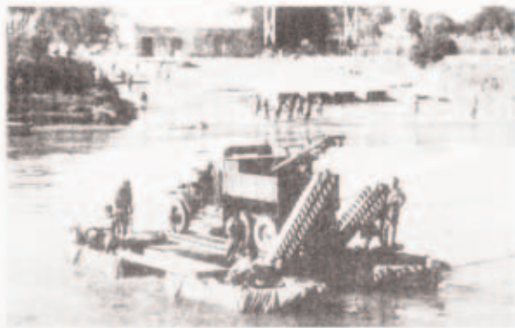
RAFT HAVING BEEN TURNED BY HAND, LORRY ABOUT TO DISSEMBLE AND GO DRIVING UPSTREAM.
