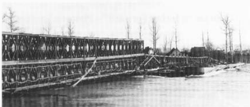
A Bailey pontoon bridge over the River Meuse in flood near Maastricht and showing the bow wave problem. Crown copyright.
