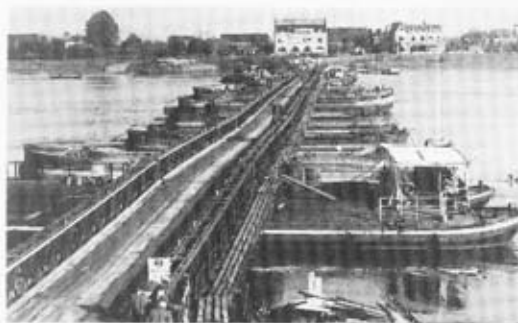
The 1100ft barge Bailey bridge over the River Rhine at Nijmegen.
