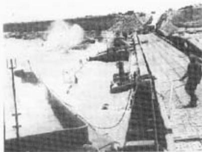
Fig. 10 Whale on L.S.T. pier damaged by drifting barges. Imperial War Museum
