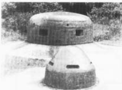
Turrets with six loopholes for machineguns and a small "bell" for infantry as an observation post.
