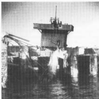
Fig. 8. Phoenix after gale with offshore walls having failed outwards. Imperial War Museum
