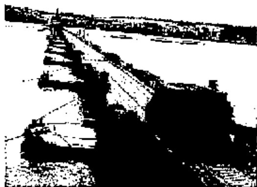
Fig. 5. Whale floating roadway in use, with concrete Beetle pontoons. Imperial War Museum
