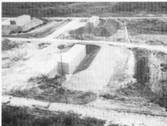
View from west of newly constructed ammunition storage sheds. Earth traverses with topsoil covering are clearly shown together with a drainage ditch illustrating the water table even though this was the "dry season".
