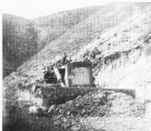
D8 working on widening Cavendish Road for tanks, looking south to Snakeshead ridge.
