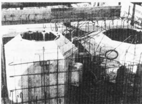
Ringstand for 8cm mortar during its building process.
