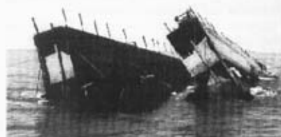
Fig. 9. Pair of Bombardon breakwaters after gale. Imperial War Museum
