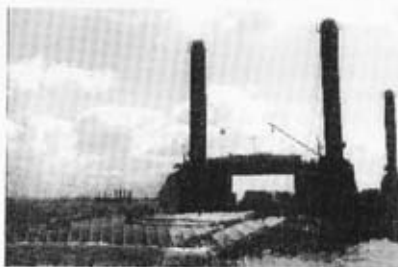
Fig. 4. Spud pontoon with L.S.T. buffer. Imperial War Museum
