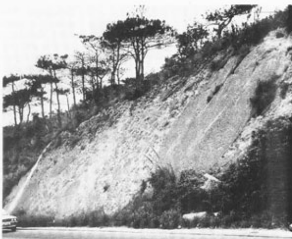
Photo 1. Slope cut through granite colluvium in Hong Kong; note striking contrast in tone, with large dark grey core stones of massive granite rock in a light grey, soft matrix of granite now weathered to sand and clay. This produces a wide variety of rock strength, and potential for confusing large boulders with bedrock during site investigation. Geological factors influence route alignment; means and speed of excavation; and slope stability. Additionally for military purposes, they influence the effectiveness of explosive cratering for route denial.
