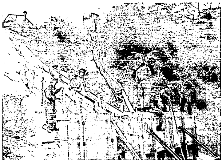
Working on the retaining wall – note the formwork on the line of the new spillway, and the gap through which it discharges.
