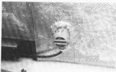
A float switch (centre) prevented the unit from being run dry. The heating elements can be seen to the left of the picture.
