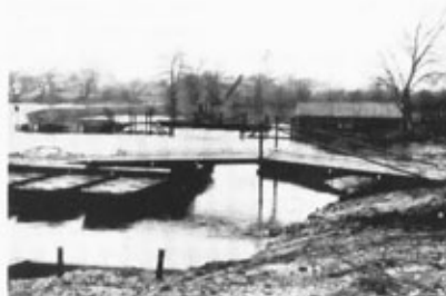
Folding Boat Equipment, known as FBE. Introduced in 1928 and developed to 9-ton capacity.
