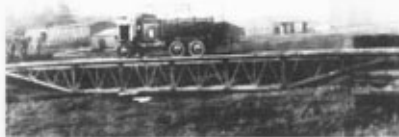
Inglis tubular truss bridge (1940 version) designed by Professor Charles Inglis of Cambridge University.
