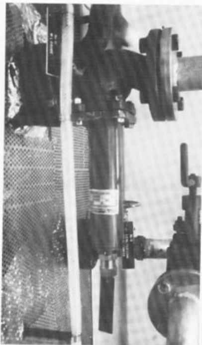
As the temperature plummeted, water was recirculated around a ring main to prevent freezing. Water pressure was maintained by fitting a mechanical pressure relief valve in the return pipework.
