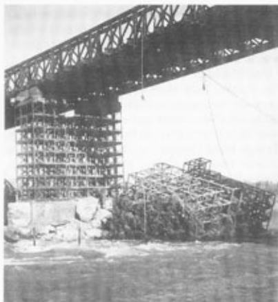
Paglieta bridge: Remains of original No 3 (north) pier with replacements.
