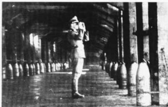
New Pier – St Peter Port showing demolition charges in position. 198 300lb French shells.
