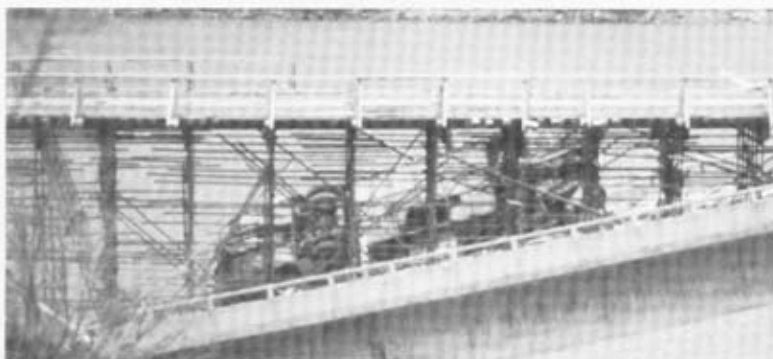
The damaged southern span and the scaffolding improvised bridge.
