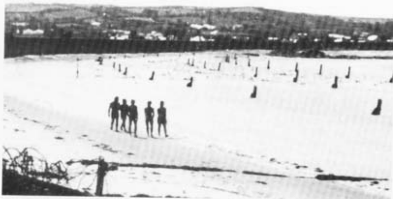
Underwater obstacles in Varon Bay – steelgirders with Tellermine on top.
