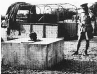
A few of the tanks were "ready made" galvanised steel. The chokra (small boy) was specially employed to go inside and caulk the leaking joints.
