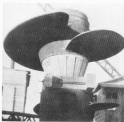
A 'screwcrete' cylinder base ready for screwing into the bed of Loch Ryan.
