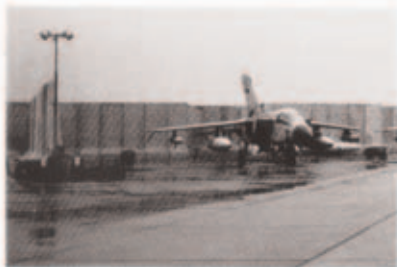
Splinter protection units protecting aircraft on RAF Muharraq
