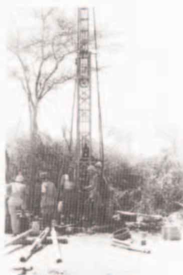
South African engineers boring for vital water supplies at Hagadera
