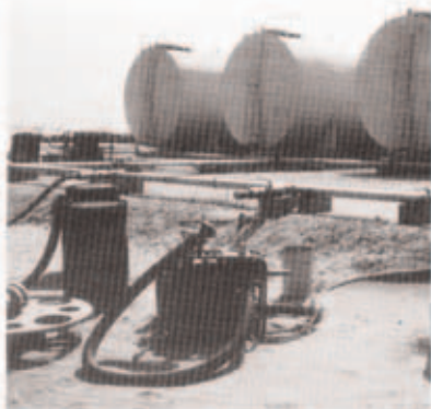
Steel storage tanks, designed, purchased, and installed for ground fuels storage in Jubayl
