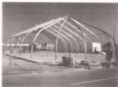
A sprung shelter being erected — Eight men for two days
