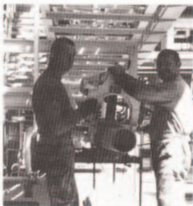
Sgt Jackson (left) and SSgt Robson making up pipe work to connect the fuel lines to the East Plant boilers
