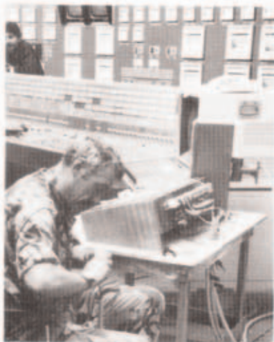
WO1 Turner rebuilding the West Plant controls. The panel beside him is all that was used to control one 300MW set.
