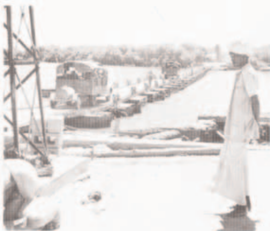
Pontoon bridge over the Juba (later swept away by a flash flood)
