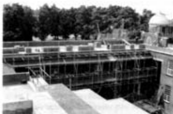
Photo 2 The Ravelin Building inner parapet wall being prepared by the contractors, Arnold and Nathan, for laying of the reinforced concrete bearing pads for the beams
