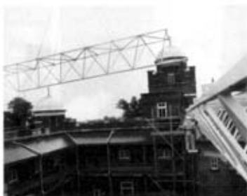
Photo 3 One of the side trusses being lowered into position in July 1990
