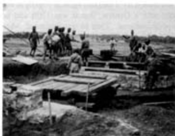
7.6.18. 2nd stage of the railway bridge. Shifting the main girder across with the aid of rollers.
