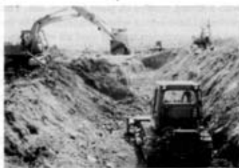
Plant working to excavate the old slot and prepare the new slot
