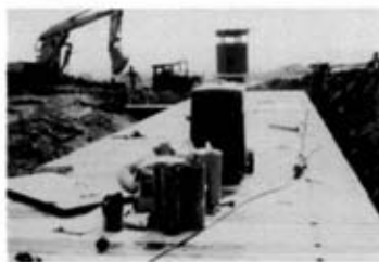
The finished roof prior to backfilling
